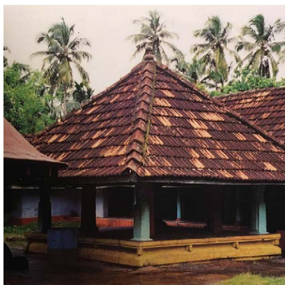
Fig.3.1.7 Sabha Mandapa Kerala, Tranquebar.
