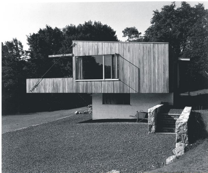
[Fig 21].Chamberlain cottage, Wayland (Massachusetts, 1940. Marcel Breuer/ Walter Gropius] [Fig 22].Breuer House II, New Canaan (Connecticut). Marcel Breuer, 1946
