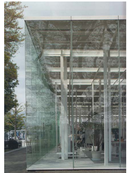
Fig.6.5.1 Kanagawa Institute of Technology Workshop . Kanagawa. 2010. Junya Ishigami
