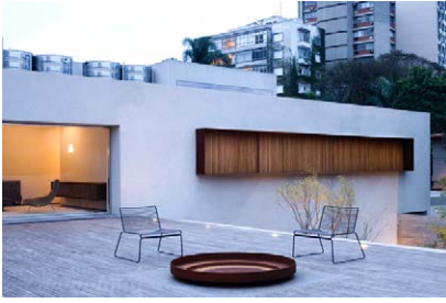
Fig.5.1.9 Chimney House. São Paulo. 2009 Marcio Kogan
