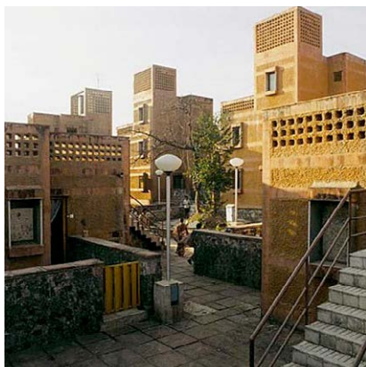
Fig.3.3.23 Sheikh Sarai Housing Project. Nueva Delhi. 1970 Raj Rewal
