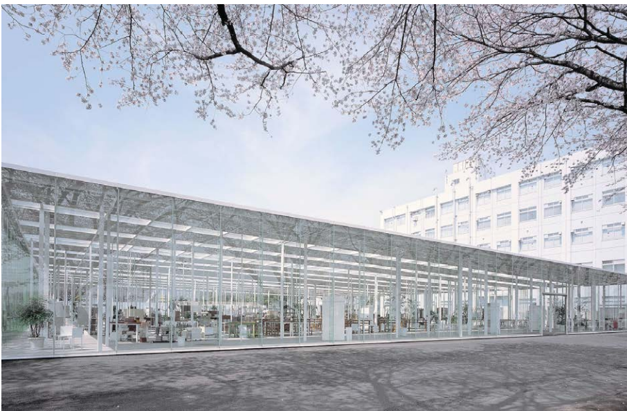
Fig.6.5.3 Kanagawa Institute of Technology Workshop. Kanagawa. 2010. Junya Ishigami
