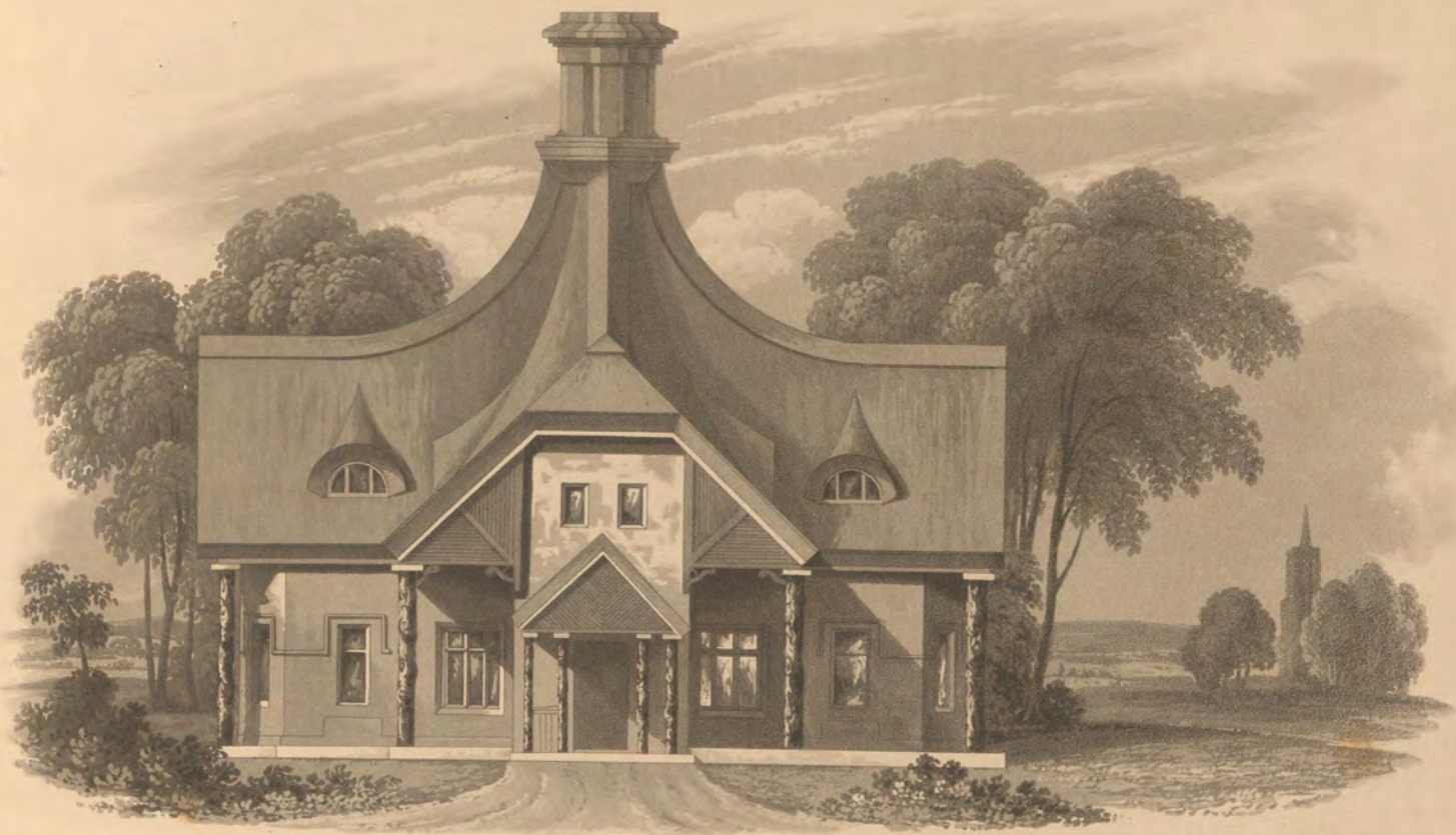
ELEVATION TOWARDS THE ENTRANCE GATES.
