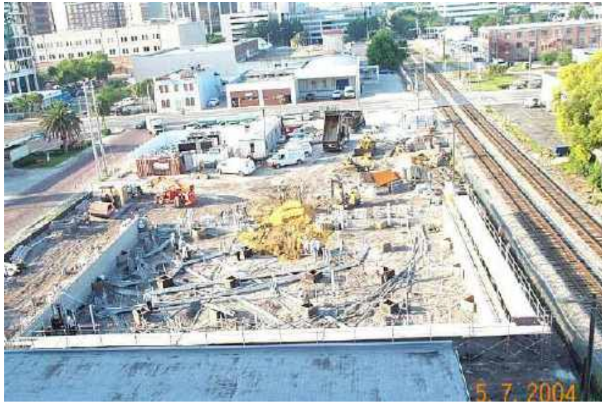
Figure 3. Installing under-slab utilities 5
