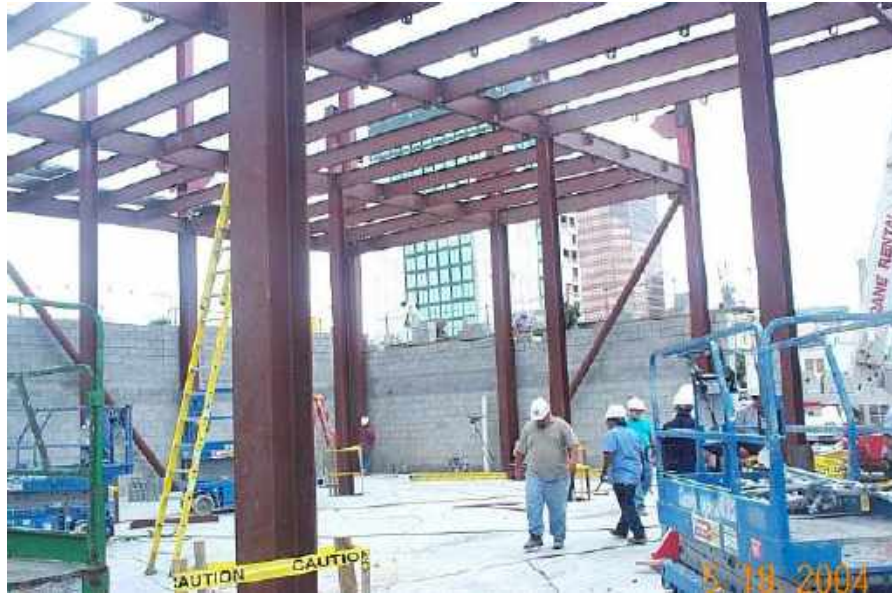
Figure 6. Structural steel beginning to take shape.
