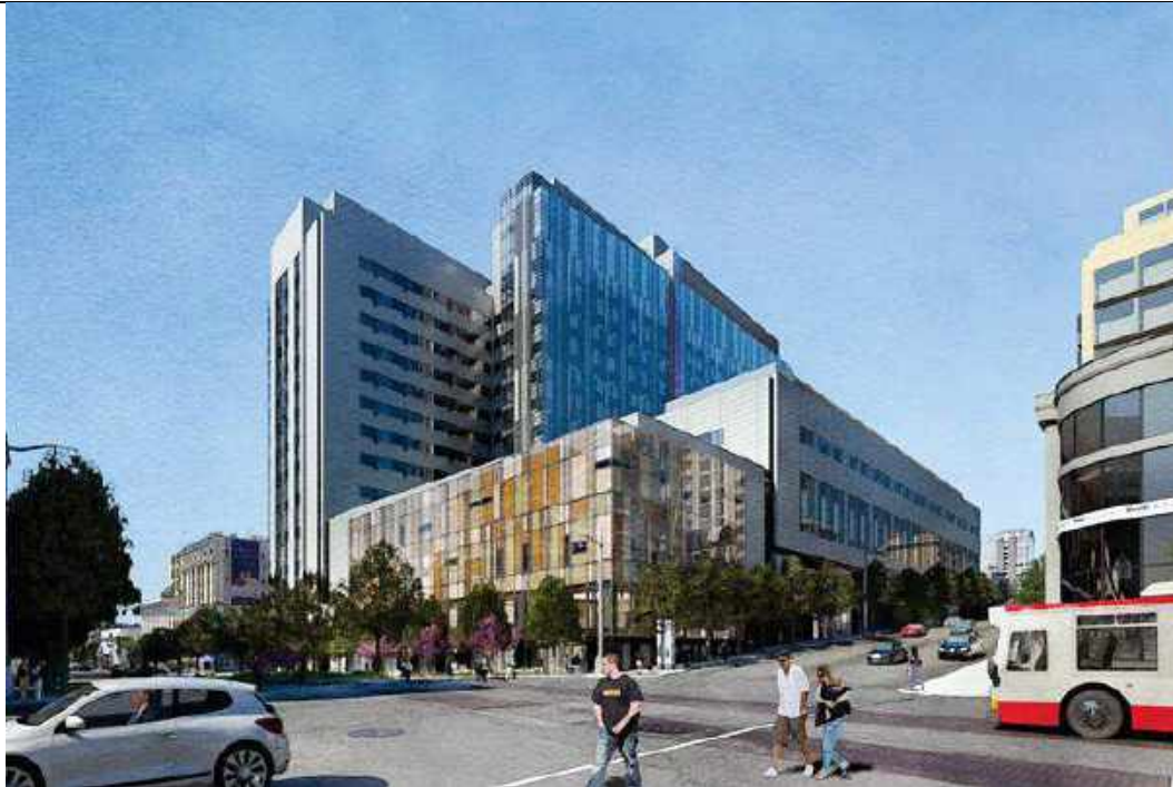
Figure 3: Cathedral Hill Hospital, San Francisco (USA)
