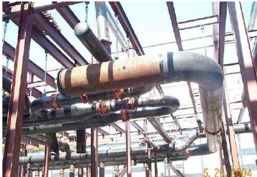
Figure 8. Pipe hoisting and installation using special crane.
