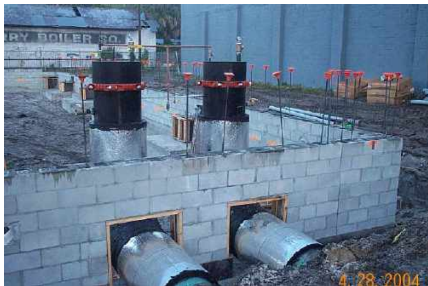
Figure 2. Step downs in the wall footer allowed for proper utilities crossing - Team decision
