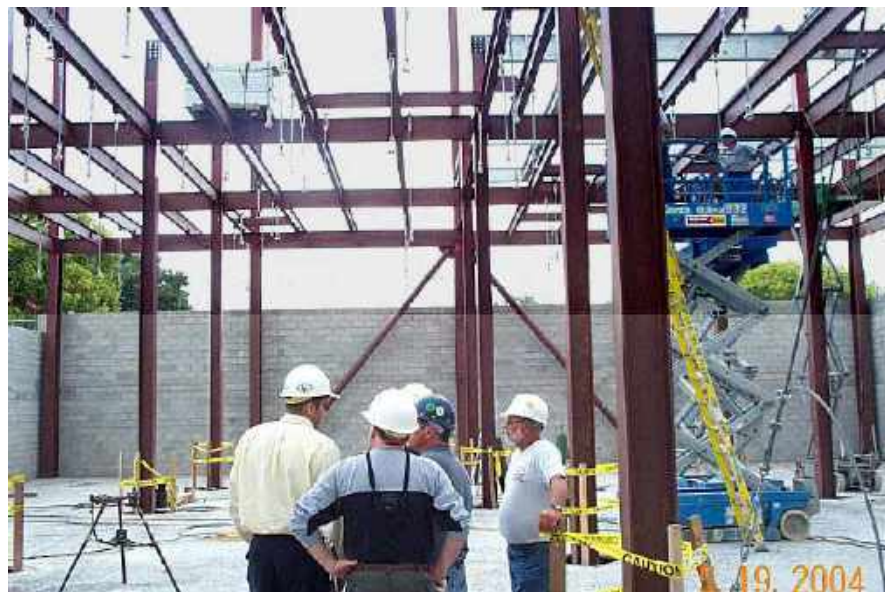
Figure 7. Hanger assemblies installed.
