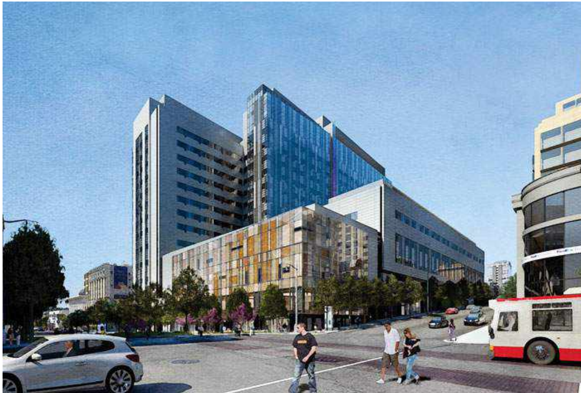
Figure 3: Cathedral Hill Hospital, San Francisco (USA)
