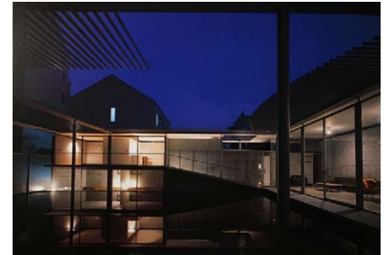
Fig.6.5 House in Tsuyama . Okayama. 1994. Toru Murakami
