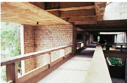
Fig.5.2.6-7-8 Indian Institute of Management , Bangalore. 1962-74 Vistas espacios in-between
