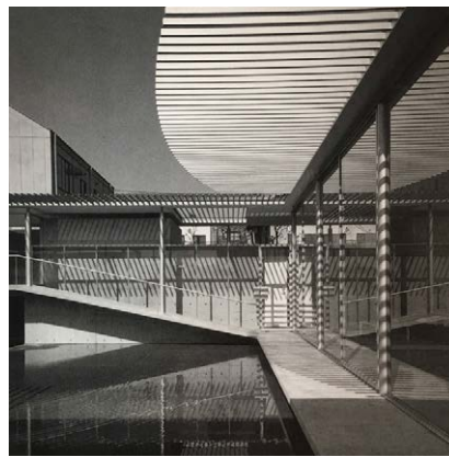
Fig.6.6-7 House in Tsuyama . Okayama. 1994. Toru Murakami
